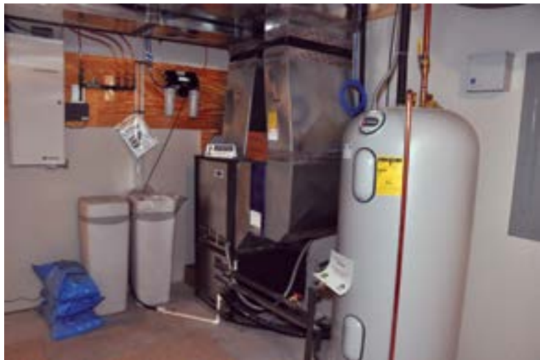
The mechanical area for one of the homes shows the geothermal equipment and a typical setup. (Photo by Merle Henkenius)
